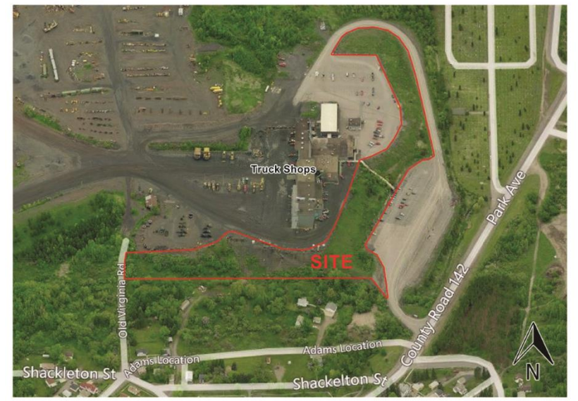
Truck Shops Embankment
