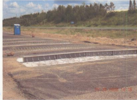
Expansion Joint Construction
