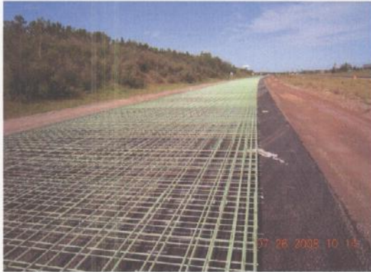
2 Layers – Reinforcing Steel
